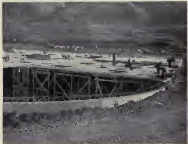
BER GASKETS on the spigot ends of the 20-foot concrete sections of the big water pipe made it water-tight (see above). At the right, columns supporting the Terminal Reservoir roof. At the bottom, covering Terminal Reservoir No. 2 with a slab roof.
